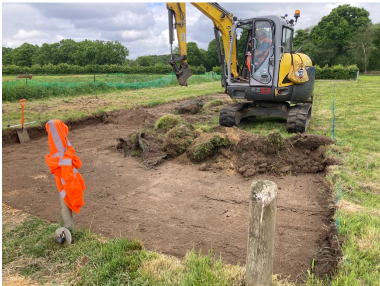
Figure 2: The top soil being removed
