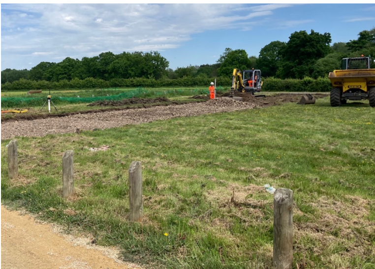
Figure 3: The recycled material being laid on top Of the geotextile material
